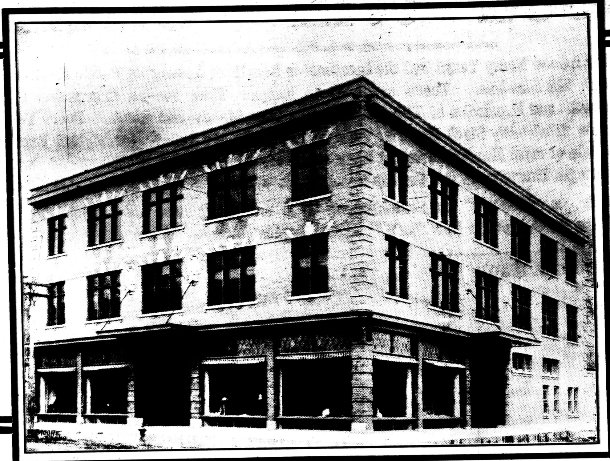
This Building has a frontage on Norfolk Street of 80 feet and on Argyle Street of 105 feet, and has four selling floors.
