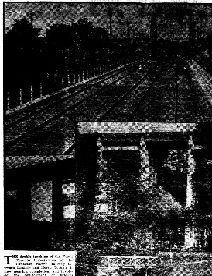
ed the replacement of bridges (known as 0.9 and 1.8) which here force had been trestles constructed of steel. Owing to the high price of successfully against steel.
