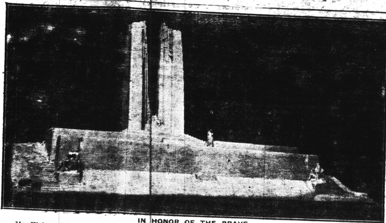
Mr. Walter S. Allward's design for a memorial on Hill 62, overlooking the Ypres Salient. This memorial was accepted by the Canadian Battlefields Memorial Commission. It is approximately 225 feet long and between 125 and 140 feet high at its highest point.
