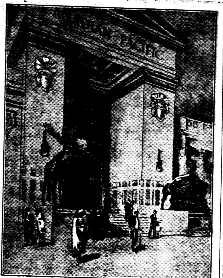
TO BOOST CANADA AT EMPIRE EXHIBITION Among the many magnificent buildings nearing completion which have been erected to house the British Empire exhibits at Wembley, next year, the Canadian Pacific pavilion is particularly outstanding.
