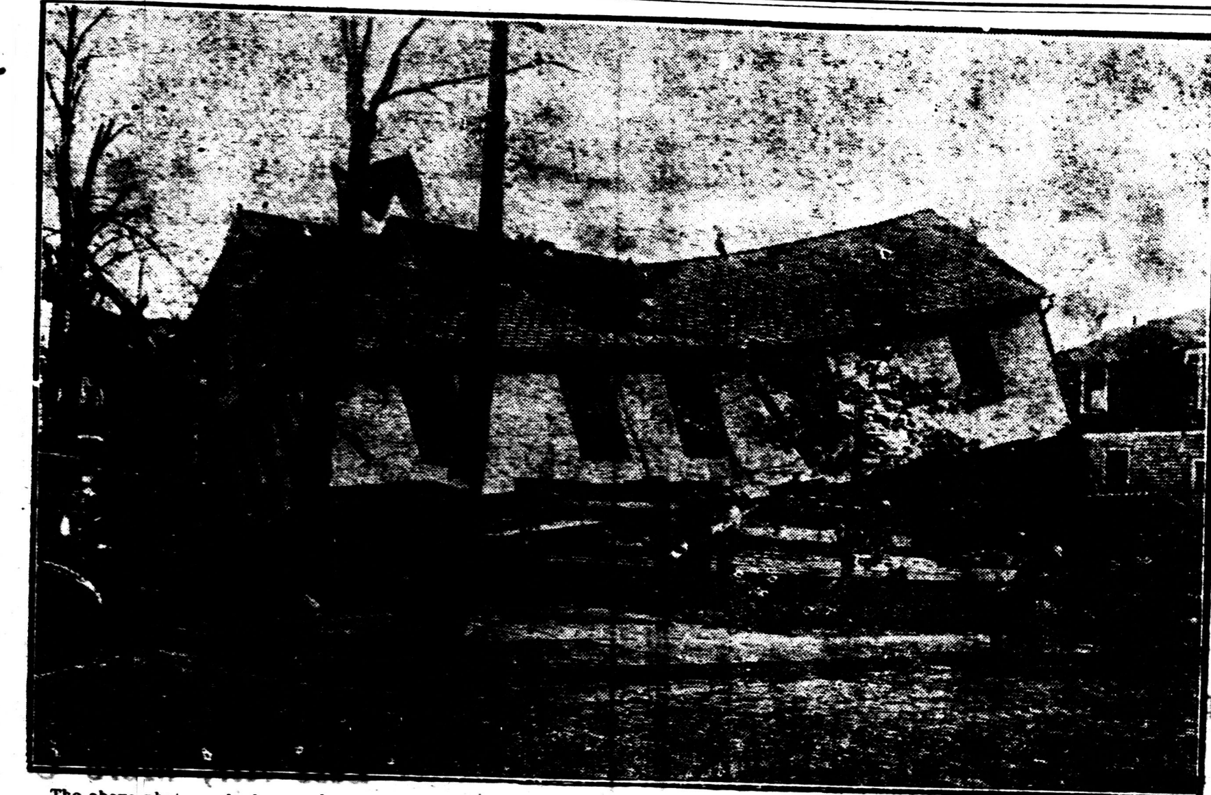
The above photograph shows a house at 6th and Washington Street in Lorain, Ohio, raised from its foundation by the tornado which resulted in the loss of probably a hundred lives while great numbers were injured and property damaged to the extent of millions of dollars.
