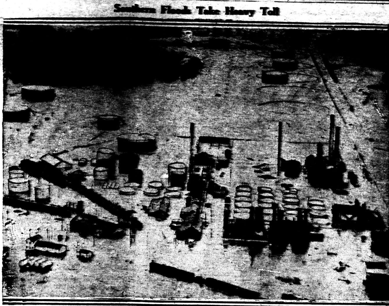
AN INTERESTING AIRVIEW OF FLOOD At Augusta, Kansas, showing the White Eagle refinery under 5 feet of water. This town was one of the worst hit by the flood.
