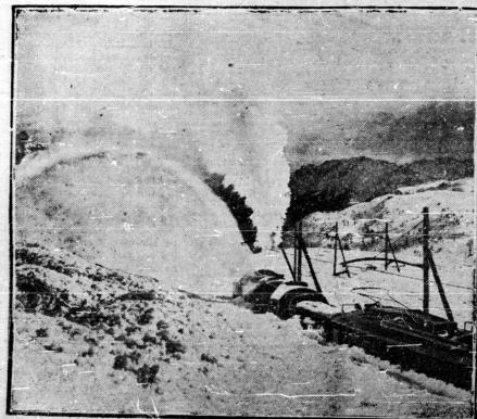
Powerful snow plow at work clearing drifts along electric railway between Tirano, Italy, and St. Moritz, Spitzerland. No matter how deep the snow, traffic is successfully maintained throughout winter on this Albine line.
