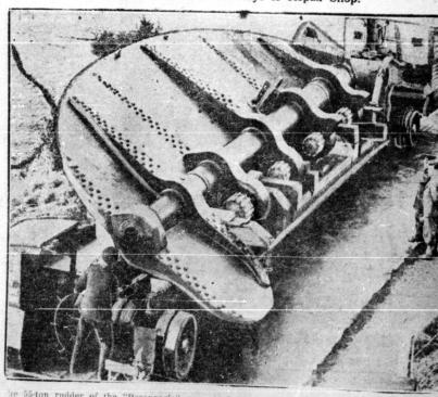
he 55-ton rudder of the "Berengaria" was carried 316 miles to Darlington, England, for 1 the trip from Southampton atter ants at front and back of the spe ally constructed, kept in touch by means of a telephone
