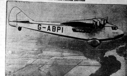
The Atalanta, first of a fleet of eight machines constructed for service on 5,500-mile route of the Imperial Airways trans-African service. The four air-cooled engines develop 1,400 horsepower and 150
