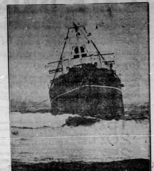
The Norwegian motorship Tai Yin which grounded at Point Reye 30 miles north of San Francisco, in a fog is shown here just before a derrick and tugs refloated it.
