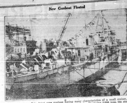
The man-of-war Erie, latest type gunboat having many characteristics of a small cruiser, pictured as she was launched in Brooklyn, N.Y., Navy Yard drydock. Displacing 2.000 tons, the staunch little fighting ship is 382 feet long and carries four six-inch guns and four anti-aircraft guns.
