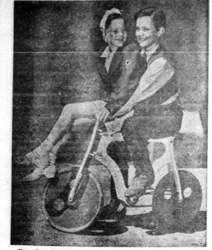
Two Los Angeles youngsters demonstrate a bicycle built of wood to meet the shortage of bikes. Three metal bolts hold the vehicle together and it runs on tires of reclaimed rubber.
