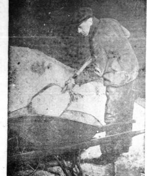
Salvaged glass is nearly 100 per cent. reclaimable. Here a workman shovels salvaged glass that has been ground into powder. Melted to a white heat in a roaring furnace, it will go to ingenious
