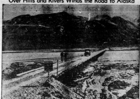
Rivers, trees, mountains and clouds form a picturesque backdrop for the highway to Alaska being built from Edmonton, Alberta, Canada, to Fairbanks by the U. S. Army. Here Army engineers have thrown a wooden bridge across a muddy stream, using more than 3000 logs. This permanent structure will be widened by the Public Road Administration sometime in the future. Alcan highway is
