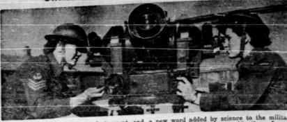
The kinetheodolite—a new instrument and a new word added by science to the military vocab ulary—records and measures the accuracy of anti-aircraft fire. It is a combination of a surveyor ulary—records and measures the accuracy of anti-aircraft fire. It is a combination of a surveyor ulary—records and measures the accuracy of anti-aircraft fire. instrument and a camera and its operation has been Army Corps who keep the instrument trained on to the target when ack-ack gunners are practising.
