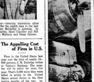
Fixing up a Flying Fortress in England, an American mechanic inflates the British "lifting bag" that acts as a jack and raises the wing of the plane.
