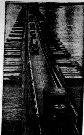
Built by Canadian Army engineers, this Bailey Bridge across the Rhine is shown shortly after it was opened to traffic. The small sign in the left foreground tells the distance that must be maintained between each vehicle so as not to overload any one portion
