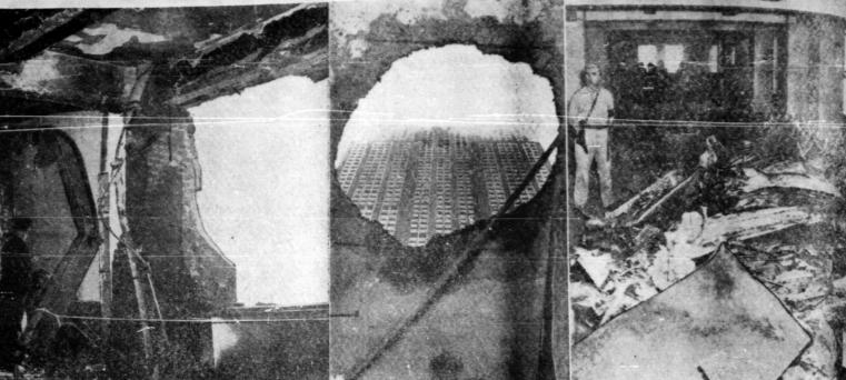
Gaping holes in the north side of the world's tailest building at the 79th floor are examined here by a New York fireman. That girder above him was twisted by force of the crash.
