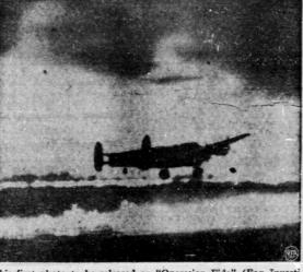
This first photo to be released on "Operation Fido" (Fog Investigation Dispersal Operations) shows how fog was articially dis-persed from RAF airfields by lines of burners on each side of main runways. In the picture, an RAF Lancaster is taking off, from clear-vision field, though fog hangs heavy up above.
