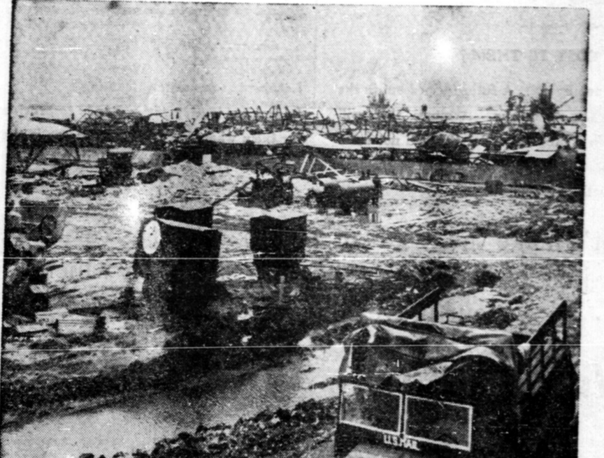
Wreckage looks like result of air raid, but was caused by fierce typhoon which struck Okinawa, demolishing U. S. Army post office and grounding many Navy ships. Only deck and twisted girders of roof remain of building as mute evidence of storm's fury.
