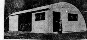
The "Quonset 24" utility building of many war uses has now been converted to the ways of peace, and especially for services on the farm. The packaged, easy-to-erect all-metal structure, shown above, manufactured at the Great Lakes Steel Corporation's Detroit plant, is described as ideal for farm tools, implements and vehicles or, with open front, as a barn for farm animals.
