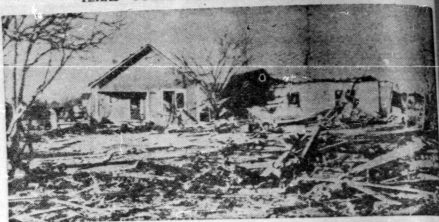
Wreckage is strewn over a wide area in Palestine, Tex., hard hit by a tornado which swept East from killing 26 and injuring 150. Remains of two frame houses are all that can be seen. Nacogdoches, Lufkin and Shiloh, Pa. were other communities in which heavy damage was reported.
