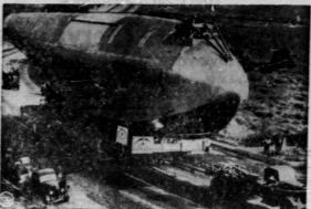
flying boat dwarfs the truck that pulls it along the highway to Ter minal Island, Calif., where the wings will be added.
