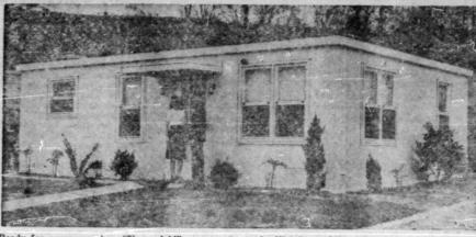
Ready for occupancy is a "Yournalaid" concrete home in Vicksburg, Miss. House was poured and allowed to set for 24 hours. Plumbing, fixtures and painting then complete the job. Home is built by a huge machine that backs over a building site, drops its huge form and is ready for the concrete. Designed by R. G. Le Tourneau of Peoria, Ill., it is expected to play an important part in solving current housing shortage.
