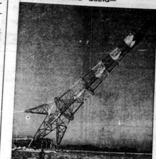
Thousands of spectators at the Ford Airport, Dearborn, Mich., were thrilled recently when they watched the 225-foot dirigible mooring mast crash down, preliminary to dismantlement for scrap. The massive steel tower was severed from its base and pulled over by cables, wound on winches of six 16-wheel tractor-trailer trucks. The mast, built in 1924 at a cost of \$250,000, is pictured above, midway in its fall.
