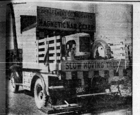
Protects Motorists' Tires-The self-described vehicle above spends the summer Ontario's major highways, removing the metal flotsam that often plays hob with car tires. Consisting of two electro-magnets, powered by a motor in the body of the the swinging beams at the rear pick up everything from nails to scythe blades. Driver's biggest problem is stopping to answer questions of curious U.S. tourists.
