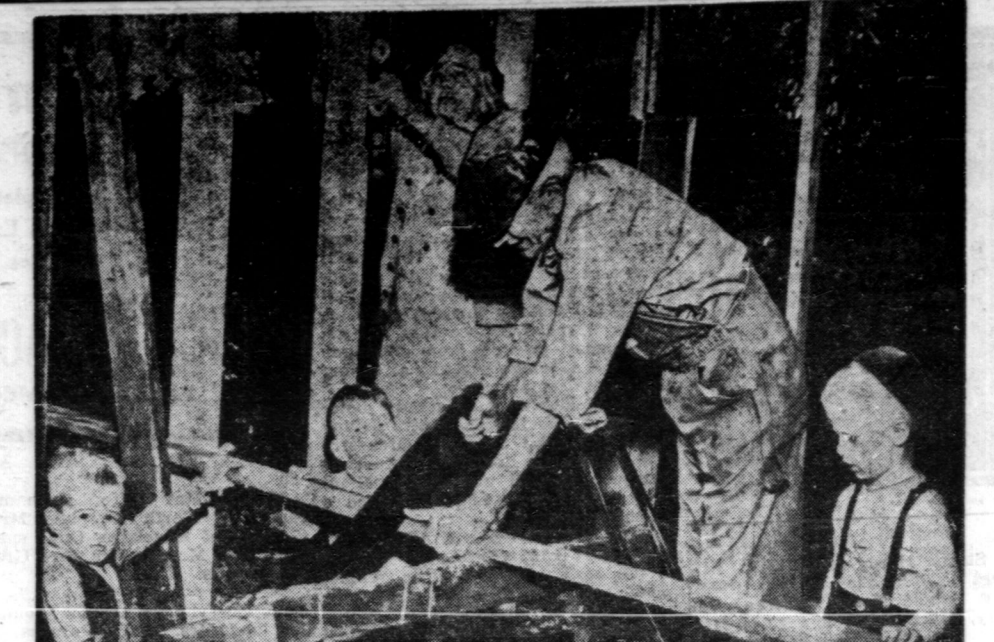
Grandpa and Grandma are "Raising the Roof"—Although this Georgia couple, "Grandma" and "Grandpa" Branran are 71 and 69 years old respectively, they didn't let considerations of age stop them from building a new house — and doing so doesn't appear to bother them as much as it does some of the neighbors who fear that one of the oldesters may slip from the perch. It's the 16th house the pair have built since 1910 which is probably some sort of a record. Some of their grandchildren are seen looking on.
