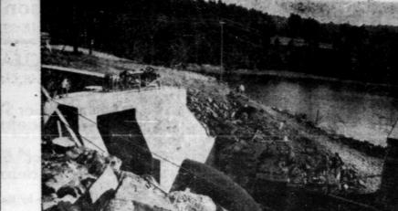
River is different from most such installations in that it will be entirely automatic in operation, requiring only the services of a caretaker. It will add 1250 horse power to the supply for the Bracebridge area with the possibility of this amount being doubled on the completion
