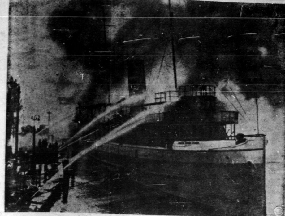
All Ashore—Fire sweeps the passenger steamer Northumberland, berthed at Port Dalhousie, Ontario, as it was about to start its 39th year on Lake Ontario. The vessel suffered damage estimated at $200,000 in the blaze which started in the engine room. It was brought under control after two hours.
