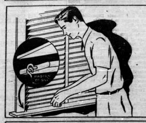
HOOKS AND EYES SCREWED INTO BOTTOM OF VENETIAN BLINDS AND IN WINDOW TILL AT BOTTOM, PREVENT BLINDS FROM RATTLING
