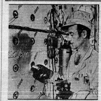
Feeding Time At Oak Ridge - A workman places an aluminum jacketed uranium slug in a fuel channel opening of one of the graphite reactors that make up the atomic pile at Oak Ridge. The ranium slugs, like the one being inserted above, weigh 2.57 pounds each and are four inches long.
