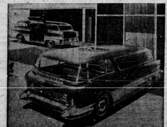
"DREAM" TRUCK WITH MANY USES —This is a drawing of a new experimental truck created by General Motors. The all-purpose delivery truck, with a 180-horsepower engine, will be called "L'Universelle." According to company officials it can easily be converted into a bus taxi, station wagon or sportsman's car. It is ten inches lower and ten inches shorter than current panel delivery trucks, yet has greater capacity. A panoramic windshield is one of the many passenger features of the unit. Part of truck's side, background, can be opened for loading.
