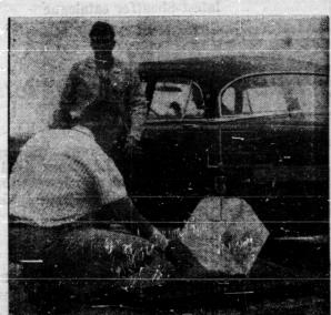
ARCTIC "LANDING"—Engineers in Marietta, Ga., show how 40-pound block of ice is mounted on outrigger attached to rear of auto and dragged at high speed over section of a plane's fuselage material to determine effect of landings on Arctic ice. Purpose: to evaluate various protective materials which could be applied to belly of the C-130 Harcules, turboprop cargo and troop carrier of the Tactical Air Command. Engineers are, from left: Lockheed Aircraft's C. D. Birmingham and J. R. Phillips.
