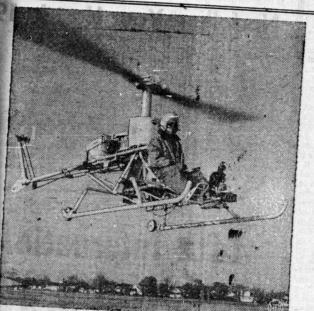
ME GIZMO - A one-man helicopter, dubbed the "Gizmo", tested. Powered by a simple two-cycle outboard motor, the eeds up to 70 m.p.h. The Gizmo is designed to serve as either ourier-liaison or tactical vehicle, permitting its use by ground es during assaults behind enemy lines.
