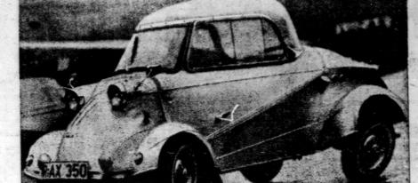
NOT TOO SMOOTH, BUT FAST — This bouncing baby car won't take any beauty prizes as it whips around a track at Brands, Hatch, England. It's a TG-500 Messerschmitt sports car, with a top speed of 90 m.p.h. and fuel consumption of 50 miles to the gallon. Has four wheels, too. (Other model Messerschmitts have only three.)
