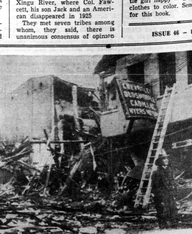
EXPLOSION IN OTTAWA — This view shows some of the wreckage in the heart of the business section of Ottawa after an early morning explosion rocked the area. No one was killed by the mysterious blast, but 35 persons were injured to some degree. The damage amounted to millions of dollars.
