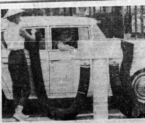
KEEPING COOL - Free air is supplied for car passengers, not tires, by an unusual cooling service offered by a drive-in restaurant. Placed in an auto window by a carhop, a flexible hose pours in cool air drawn through underground ducts from a 30horsepwer air conditioning unit. A control in the house outlet permits motorist to adjust the amount of cold air piped into the Who Will Tackle This?
