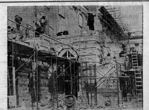
BIG BOYS' BUILDING BLOCKS - Covered since about 1822, arches once a useful part of the Washington Capitol are revealed during extension of the east front of the building. They had been hidden by a stair well. Each block of stone has been numbered according to a master plan. Arches may be set up elsewhere some time, perhaps as a historical monument.
