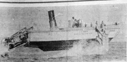
GOES LIKE A HALOBATES - You can't liken the strange craft, above, to anything else in the water. It's a "Halobates," a hydrofoil-equipped craft powered by a gas-turbine engine.
