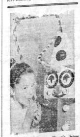
CAMOUFLAGE - Here's how some ingenious person has tricked-up a new oxygen dispenser to make its use attractive to small try. Clown's left "eye" is a pressure gauge that moves when oxygen is dispensed; hose unit is given o candy-striped effect with tape, and a party hat screens the mixer mechanism.
