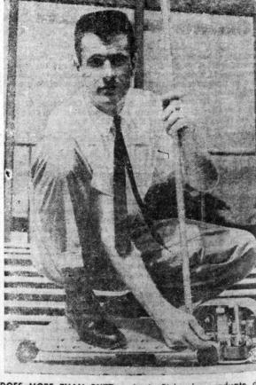
DOES MORE THAN BUZZ - Louis Richards, graduate design student at Illinois Tech., has harnessed the gnatty buzz of a 1.32 h.p. model aircraft engine to ground transportation. His "Skeeter," an 18-inch-long aluminum platform on wheels, carries its passager in two-footed somfort at about 12 miles an hour, three times the speed normally made by a pedestrian. Highly maneuverable, the 12-pound device folds into a canvas carrying case.
