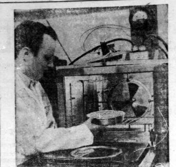
REAL "COOL" COOK - Installing a fan unit in the oven is a real "cool" experiment for Frank D. Borsenik, laboratory engineer. Fan circulates the heated air more efficiently, and a roast can be cooked at 250 degrees Fahrenheit. How that cheesecake will cook remains to be seen.
