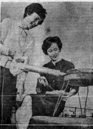
HOT AIR GUN - Valerie Druker, left, lights a barbecue fire In jig time with a flameless, hot air gun in London, England. The gun has an electric element and a fan. It heats air to eight times boiling temperature and blows it out the nozzle. No paper, kindling or chemicals are needed. Mary West waits for a good fire to pop the steaks on.
