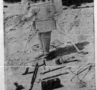
MOON SUIT - Little house with legs was designed for the moon. Republic Aviation designed the suit to provide the moon explorer with a livable atmosphere. Demonstrator puts down tripod withdraws legs and sits on a small shelf to rest. While the model is experimental, designers believe the same fundamental concept will be practical for the first moon men. Tools
