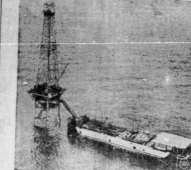
OIL FROM, THE OCEAN - Farthest offshore oil drilling instullation is this platform 70 miles off Louisiana in the Gulf of Mexico. Built by CATC (a group of four oil companies), it rises 229 feet above the water, which is 180 feet deep at this point. The tender alongside the rig holds the pipe and other drilling gear and provides eating and sleeping quarters for the crew. Platform at aft end is for helicopters.
