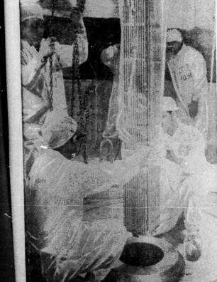
RESS HEHEARSAL - Wearing plastic "surgical" suits to ximum cleanliness, workmen practice loading a mulated fuel cell aboard the nuclear merchant ship Savanhas the cell aboard the nuclear merchant ships have the cell is identical to the real cells, 32 of which will be loaded to power the ship at a later date. The actual "fueling" will take about four hours.
