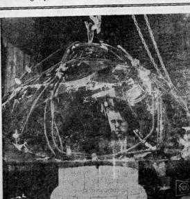
LOOKING GLASS - From this single, huge chunk of glass -48 inches thick and weighing 4,000 pounds -- will come a cision-finished telescope mirror 84 inches in diameter and 13 inches thick. The glass blank, is destined for a telescope at the University of La Plata, Argentina. When finished in 1962, the telescope will be the largest in the Southern Hemisphere. A company official inspects the glass before it moves into the melting oven.
