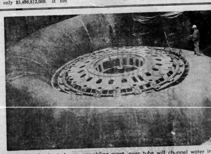
WHOPPER—Steel spiral case resembling giant inner tube will channel wat 242 feet high The water which backs up will create a lake 250 miles long.
