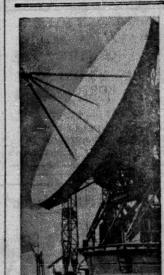
ON GUARD!-This giant, 68fuot radio-telescope is being used by scientists of the radio astronomical station of the U.S.S.R. to carry out observations of the moon, solat systems, planets and radio nebula It is near Moscow.
