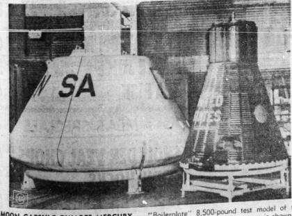
MOON CAPSULE DWARFS MERCURY - "Boilerplate" 8,500-pound test model of the Apollo Command Module, which has been planned to take men to the moon, is shown at spacecraft center where it will undergo land and water tests. National Aeronautics and space Admirish the Mercury spacepace Administration photo shows relative size in comparison with the Mercury spaceraft, which took John Glenn and Scott Carpenter on their orbital flights.
