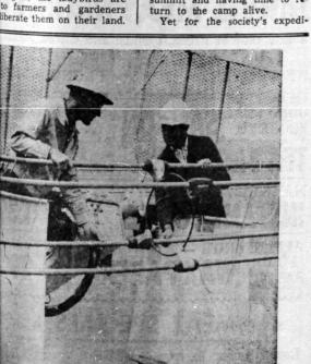
HANDED - These transmission men demonstrate handle 775,000 volts with their bare hands. Scene part of a recent series of work tests on voltage lines th showed the feasibility and safety of performing work day's high levels of voltage
